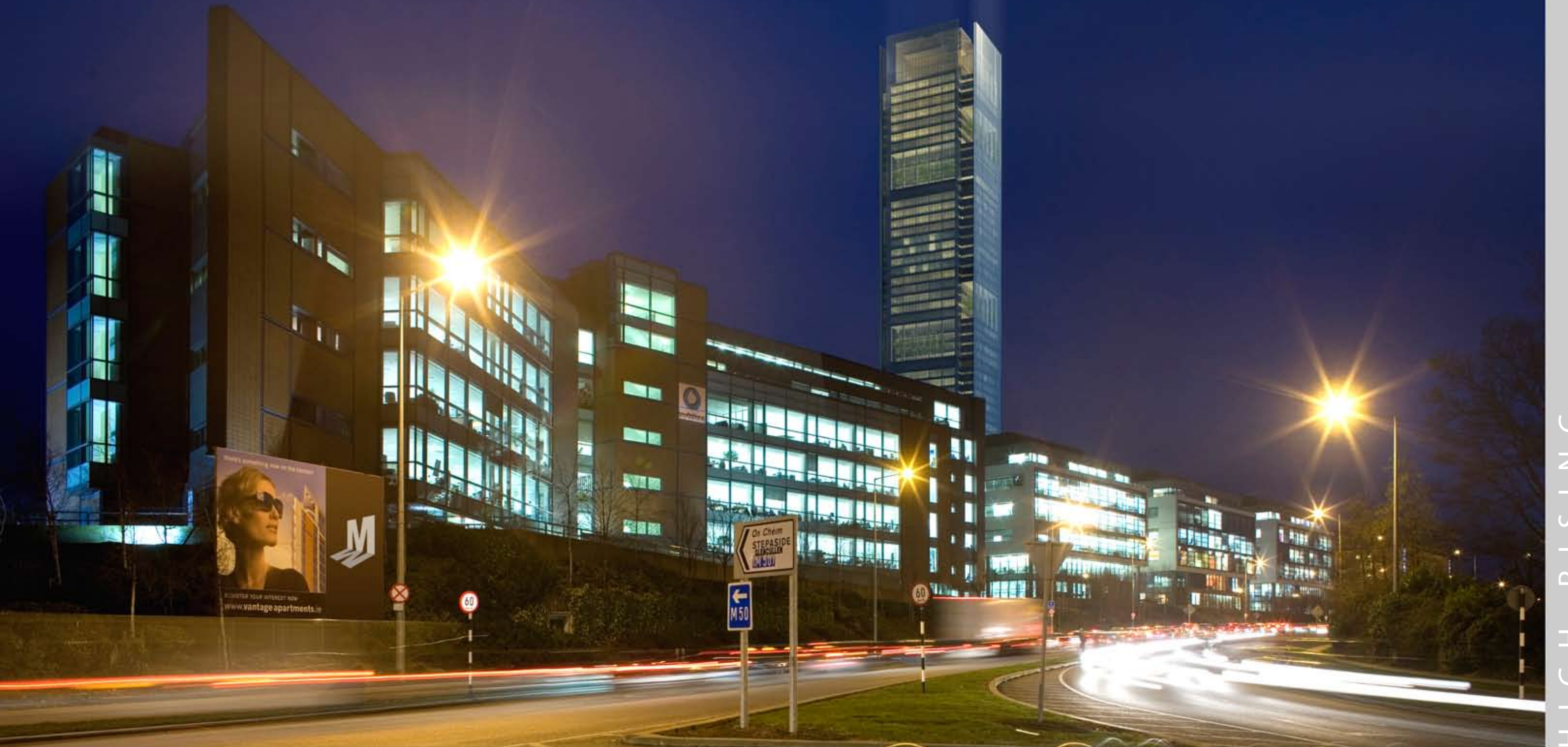
TARTAN TOWER BLOCK T-CENTRAL PARK, LEOPARDSTOWN.
